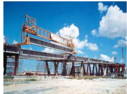
**Cast-in-Place Segmental Balanced Cantilever Bridges**
