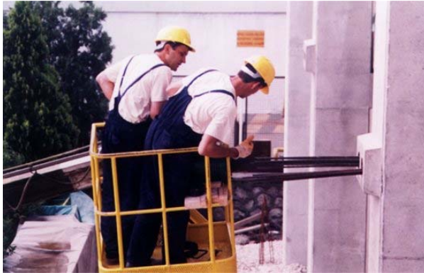
Figure 1.4 Post-tensioning process after the beams are placed in a building project in Turkey with ductile connections of jointed systems.
